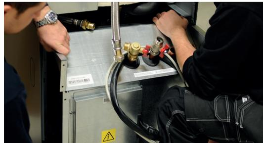
4. Pull the cooling module by first lifting the front edge slightly with the carrying handles.
