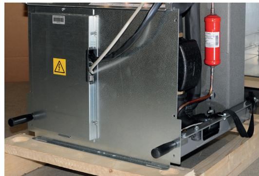
6. Lift the cooling module into the product using the carrying handles and shoulder straps. Remove the carrying handles and reconnect the power cable, hoses and screws.
