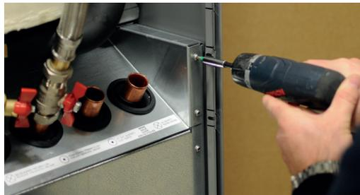
3. Unscrew the cooling module's screws.
