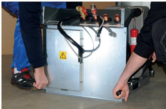
5. Lift the cooling module using the carrying handles and shoulder straps.
